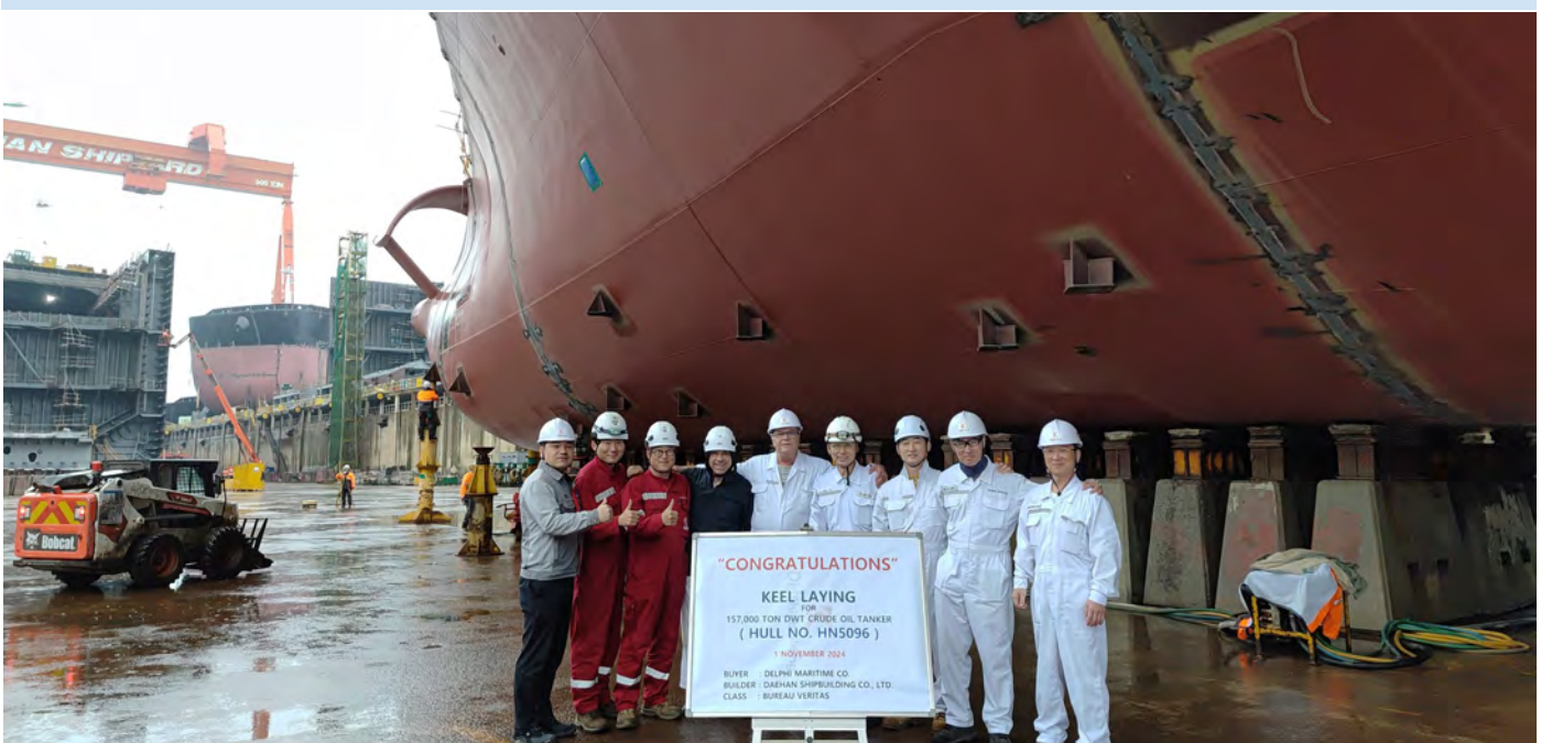
Keel Laying of M/T Energy Dione
