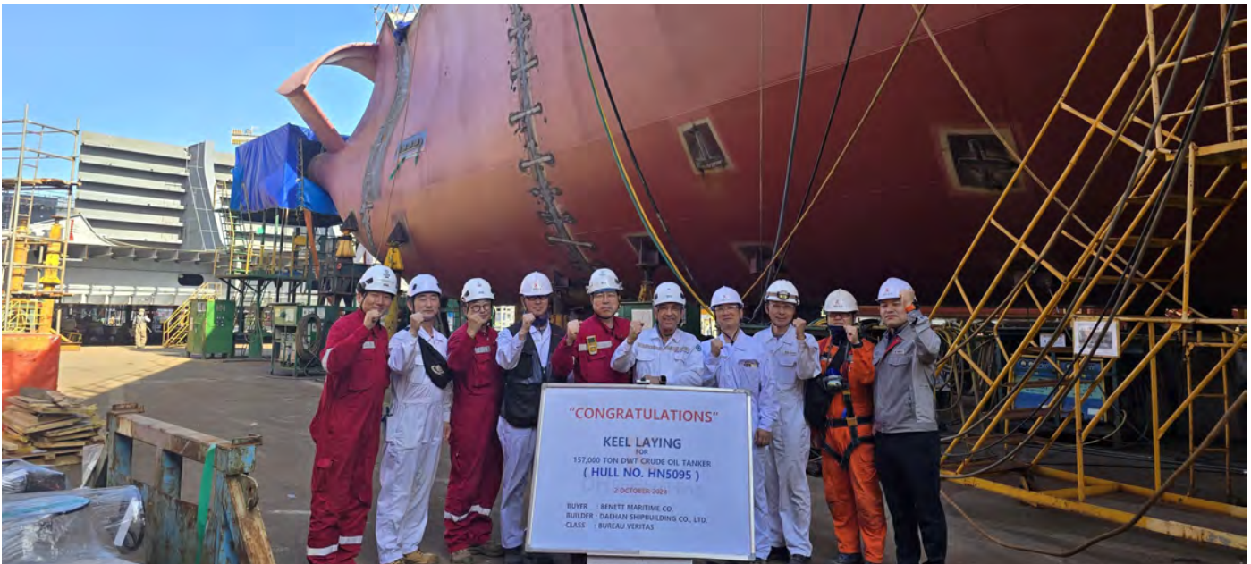
Keel Laying of M/T Energy Delos
