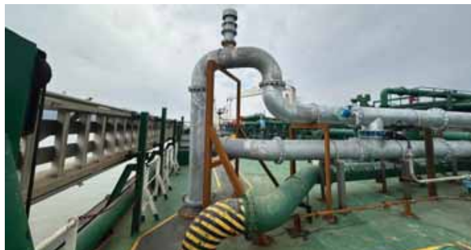
BWTS Piping on Deck
