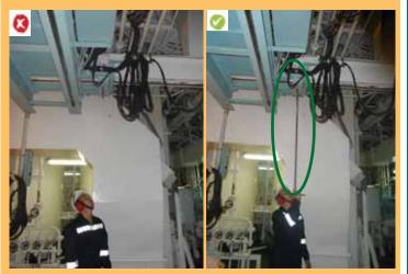
What happened: A remote key was manufactured in order to reliably secure the machine crane in place and prevent unintentional movement.
