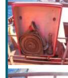
pened: During weekly inspection of the FFE, it was found that the cover of a fire hose box was missing.
