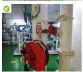
What happened: The fire hose located near the ECR was not connected to the fire hydrant.
